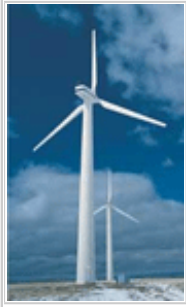
A wind turbine
