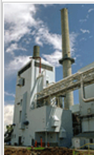
A biomass power station
